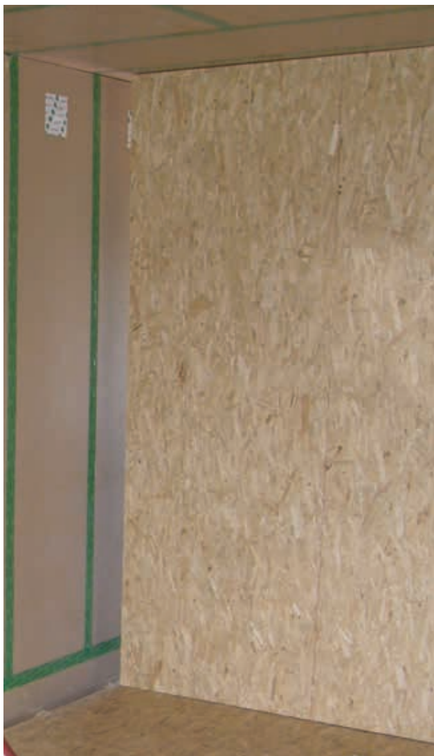
Image17: Example of wood house applying OSB Airstop boards when the structure is designed in a way to reduce the number of construction connections between the internal load-bearing walls and the sheathing to the minimum with a possibility to control the main airtight layer during the whole time of construction.
