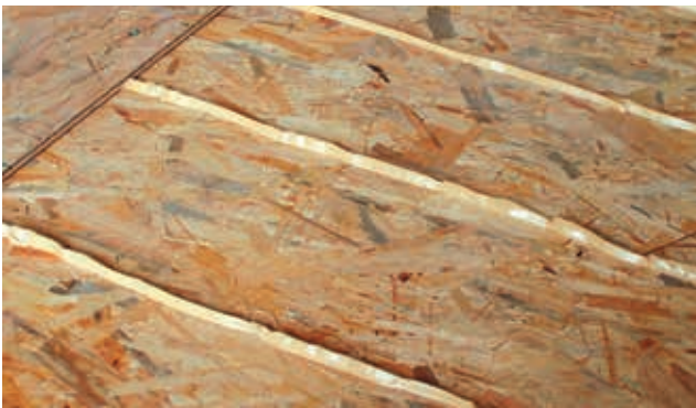
Image13: Gluing OSB boards with gun
